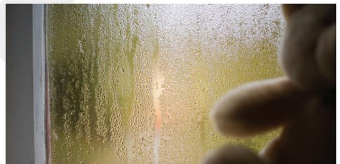
In summary, condensation is a climatic condition that is caused by water vapor changing back into a water form. Glass does not cause the condition, therefore it is not considered to be a product fault.
